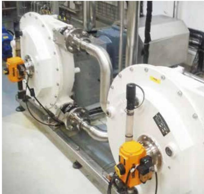
High maintenance diaphragm, rotary lobe, or progressive cavity pumps are unable to match the dependability of Bredel hose pumps in heavy duty applications.
